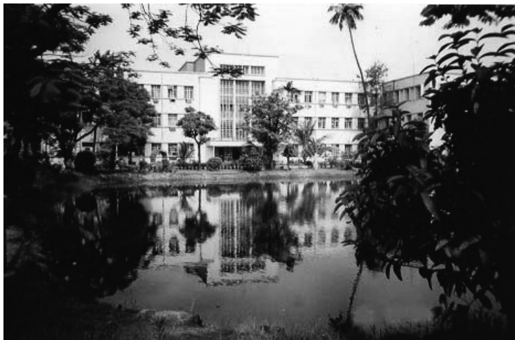
The new building of Indian Association for the Cultivation of Science in Jadavpur, Kolkata
